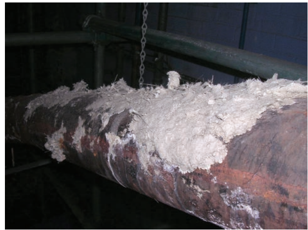
▲ Figure 1.5 Asbestos in poor condition
