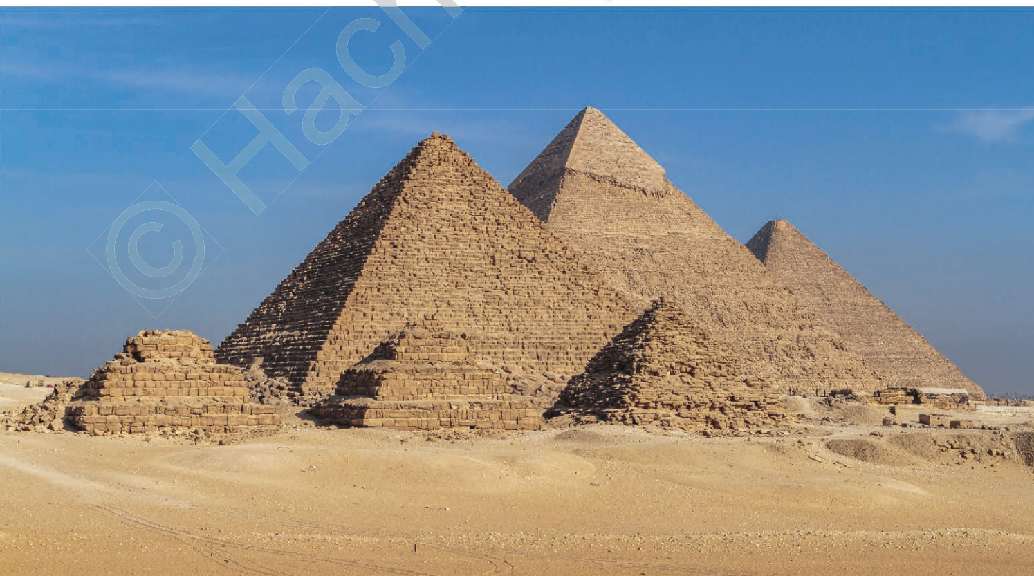
Figure 1.5 Neolithic: Egypt. Pyramids at Giza, c. 4500 years ago. Nile stone and limestone. Khufu Pyramid: 230 x 230 m base, 146 m tall.
