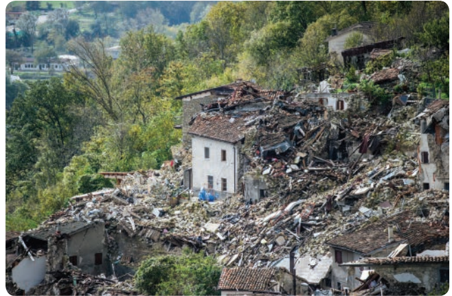
A: Earthquake damage in Central Italy in 2016
