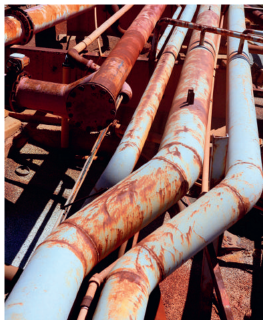
Figure 1.1.11 Corrosion on industrial pipes
