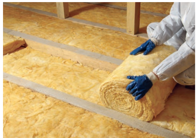
▲ Figure 3.4 Loft insulation
