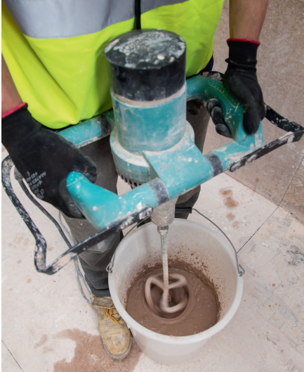
▲ Figure 3.21 Mixing with a drill and whisk
