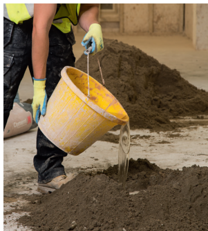
STEP 7 Pour the water into the middle of the pile of materials.
