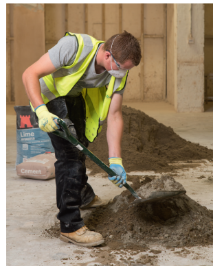
STEP 3 Mix the materials dry (without adding water).
