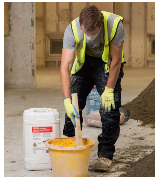
STEP 6 Mix the plasticiser into the water.
