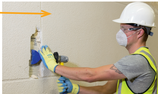
▲ Figure 3.14 Hacking a surface
