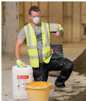
STEP 5 Measure the correct amount of plasticiser needed to improve workability. Add the plasticiser to the water.
