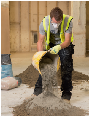
STEP 2 Next, place the materials into a single pile.
