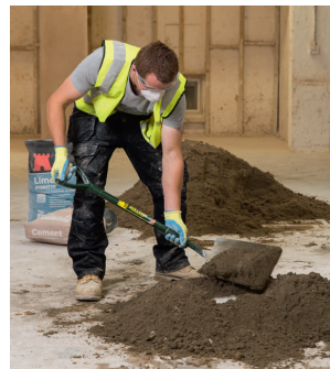
STEP 8 Using a shovel, pull the dry material slowly towards the centre, into the water.
