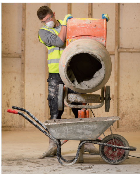
▲ Figure 3.19 Mixing with a drum mixer
