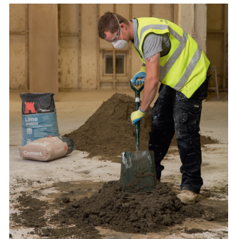
STEP 9 Mix and turn the material. The longer you turn, the better the mix.
