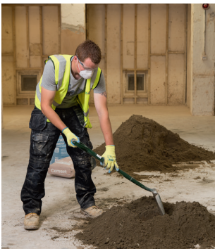
STEP 4 Once the materials are mixed, make a dip in the middle of the pile.
