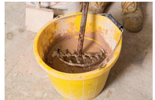
▲ Figure 3.20 Mixing with a plunger
