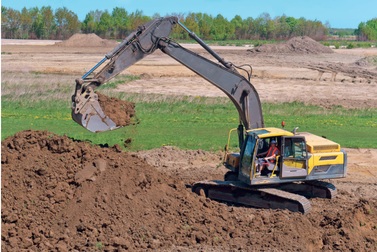
▲ Figure 2.3 Removing topsoil
