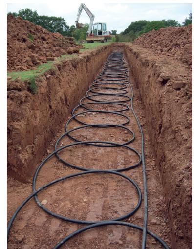
▲ Figure 1.15 Slinkies being installed in the ground
