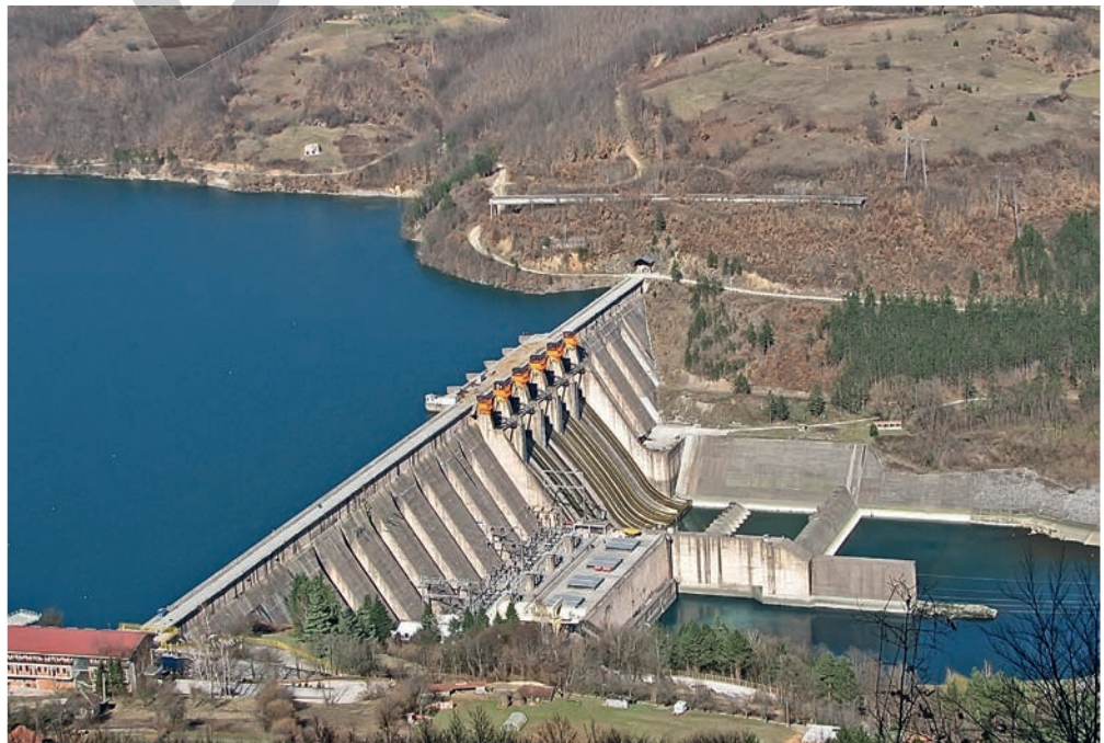
Figure 1.2.7 Hydro-electricity channels water through turbines to turn generators producing electricity
